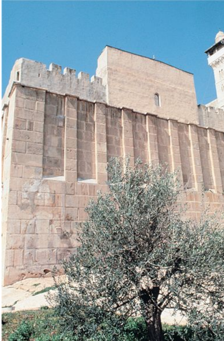
Herodian structure built over the Cave of Machpelah, Abraham's burial place for Sarah.
